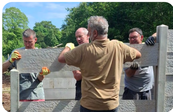
A team of High Constables helped construct new compost bays.
